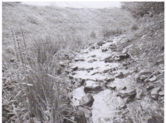
Rock Rolls used with Coir Rolls on a cobble bed stream
