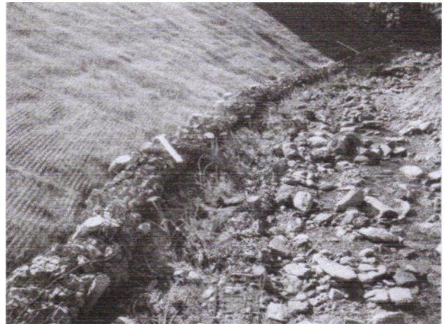
Rock Rolls used with Coir Rolls on a cobble bed stream
